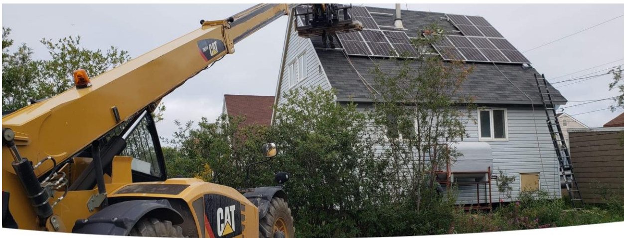
Pictured: Installation of PV Solar on home in Inuvik
